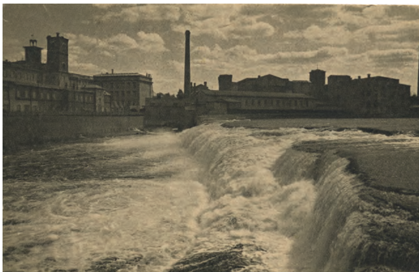
Fig. 2. The Narva waterfall was the largest in Europe with maximum flow extending to 2000 m 3 /s (before the construction of hydropower plant). Postcard from 1930s.
